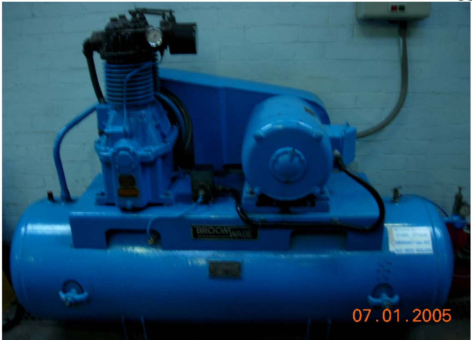
The air compressor in Sussex boiler's house
